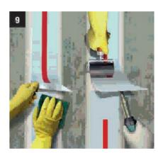
Connect tape ends by hot air welding. Prepare the welding area by roughing the surface by scotch brite or sand paper. Overlap 40 - 50 mm.
