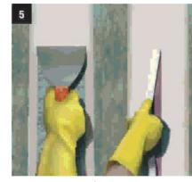
Apply the Sikadur®-31 C adhesive on the left-hand and the right-hand side of the joint. Then remove masking strip.
